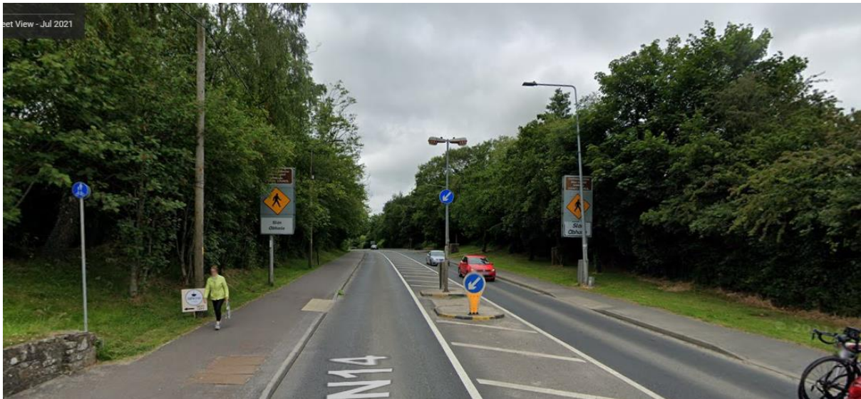
Figure 5: N14 Letterkenny Road Proposed Site Entrance (to the right just at grey car)
