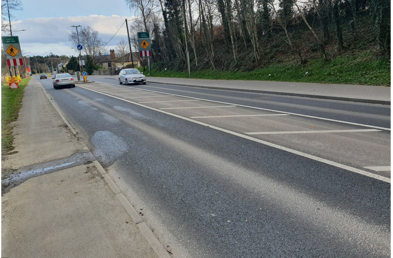
Figure 2 – Existing road markings at proposed junction location
